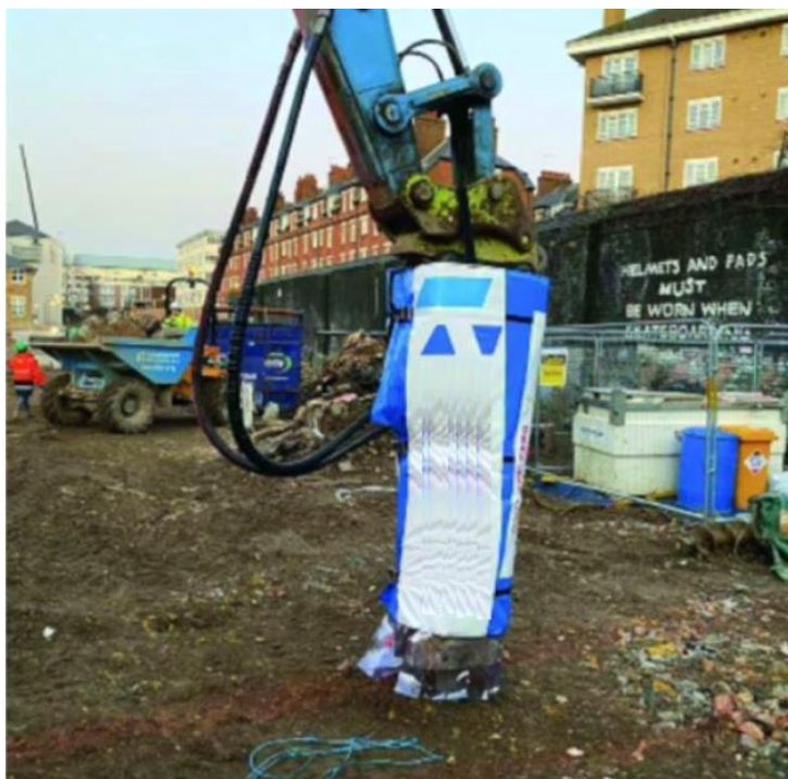
Figure 8 Example Acoustic Shroud Around Breaker
